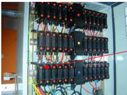
Hot terminal in a fuse box causing intermittent lighting problems detected by thermography
